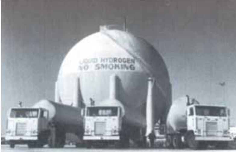
Figure 20. A picture of a liquid hydrogen tank, along with several liquid hydrogen delivery trucks (Photo obtained from NASA's website at www.nasa.gov ).
